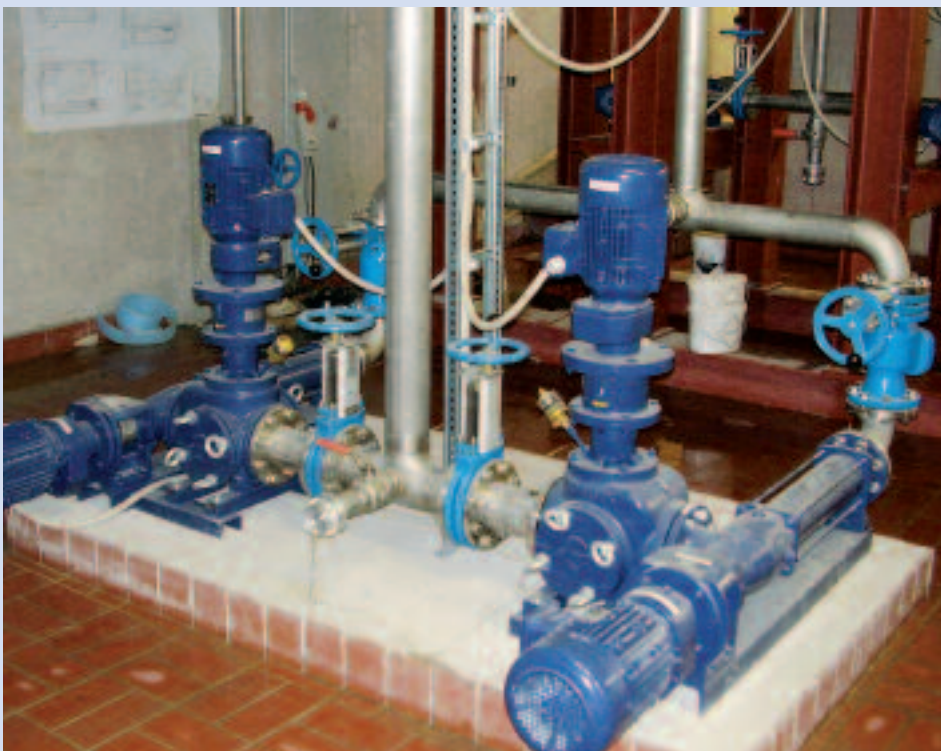
Flotation-sludge pumps
